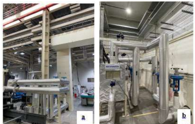
Figure A.2.21: Actual site photographs of interconnecting piping system a) Termination to HHFTF b) Origin of pipes from EHCL.
