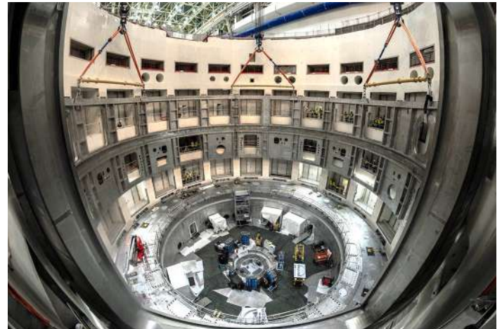
Figure B.1.3: Cryostat (Base section and Lower Cylinder) installed in Pit at ITER-Site.
