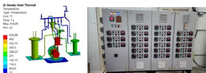
Figure A.2.9: Steady-state thermal analysis of Tin-Lithium Loop (Left). PID based temperature controller is energized and ready for integration with Tin-Lithium Loop (Right).
